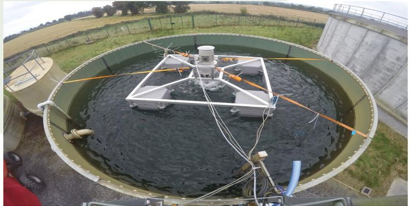
**Picture 1:** An example of some of the microbubble technologies being used by MOREFISH. This unit produces microbubble in the 50-500µm range through mechanical shearing.
